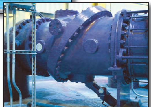
Tilted Disc Check Valve with Bottom Mounted Oil Dashpot.
