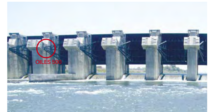
Maheshwar Dam (India), Radial Gate
