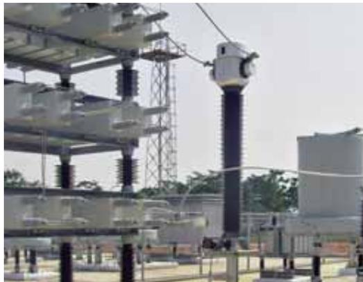
2. 245 kV Current transformer protecting capacitor bank (India).
