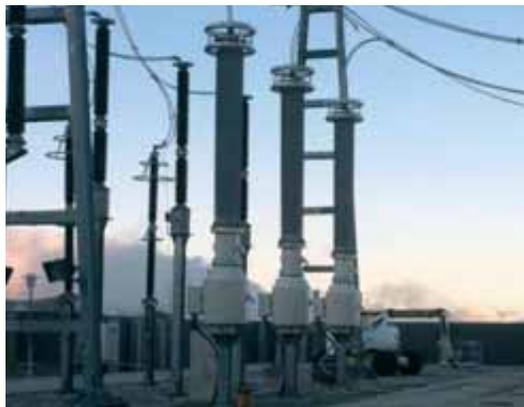
4. 420 kV Inductive voltage transformer. R.E.E. (Spain).
