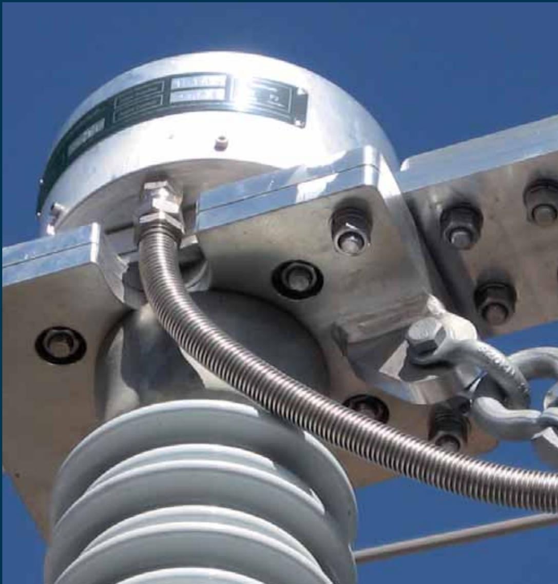
› Optical current transformer SDO OCT.
