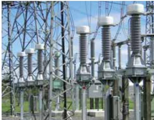
2. 123 kV Inductive voltage transformers. Transpower (New Zealand).
