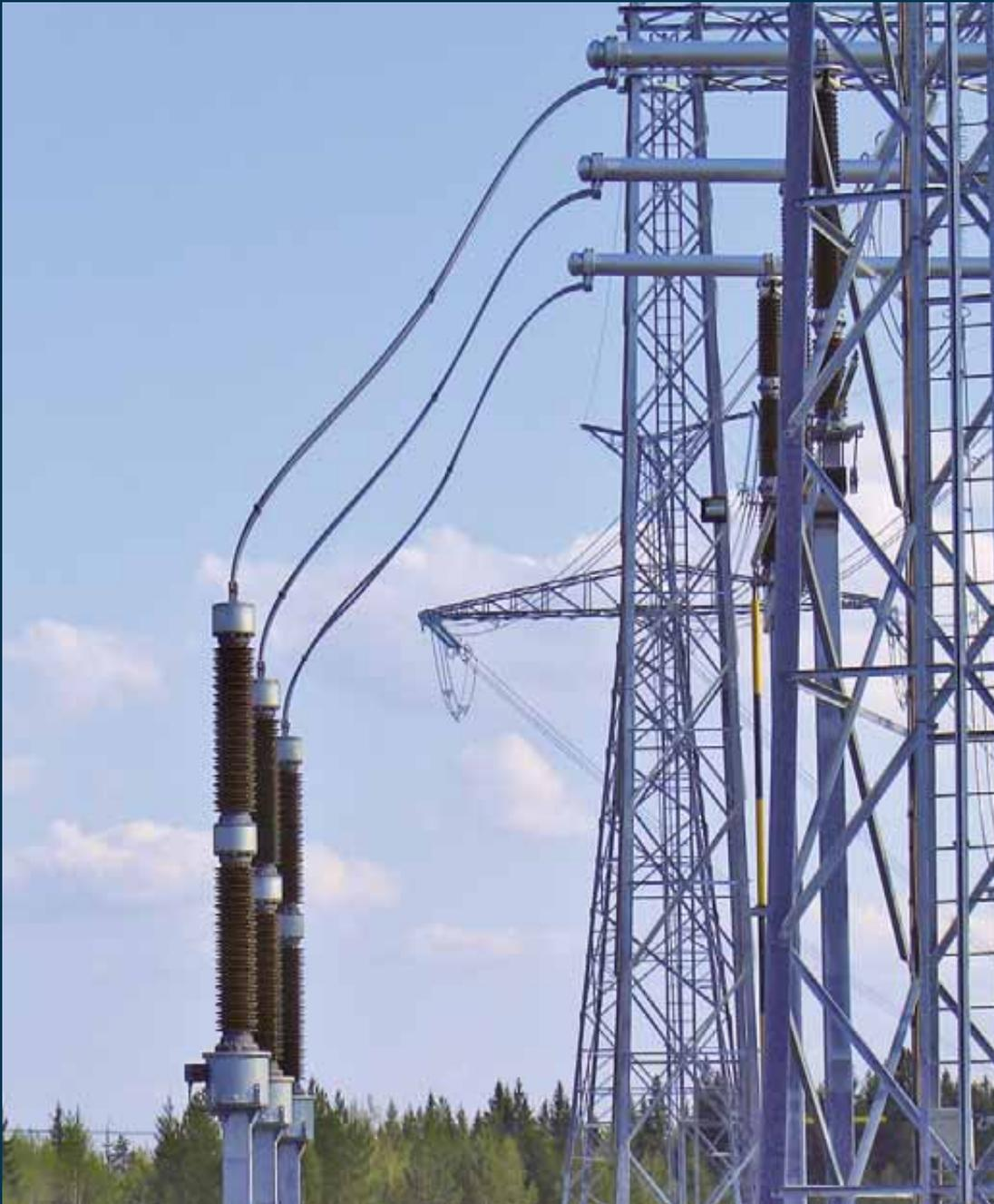
› 420 kV Capacitive voltage transformers. Fingrid, Visulahti (Finland).
